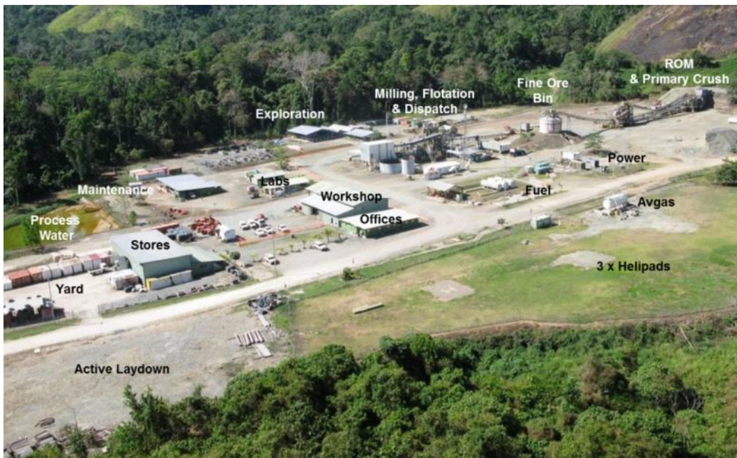
Figure 3. Oblique view of Process Plant and office infrastructure area (circa 2012)
