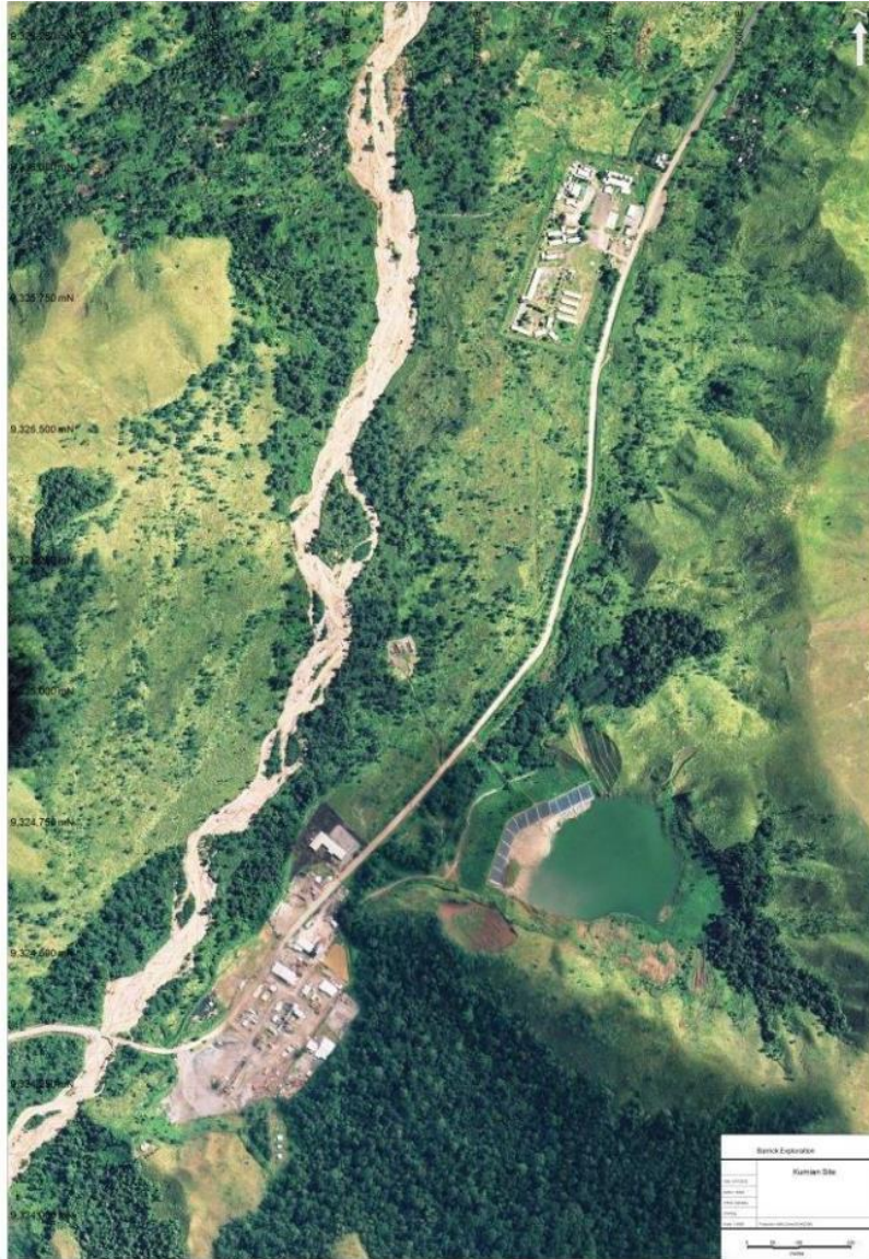
Figure 6. Aerial view of Process Plant, Tailings Storage Facility and Accommodation Camp (circa 2009) Source: Barrick 2012
