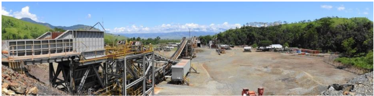
Figure 34: Photograph of the Crushing Circuit (2012)
