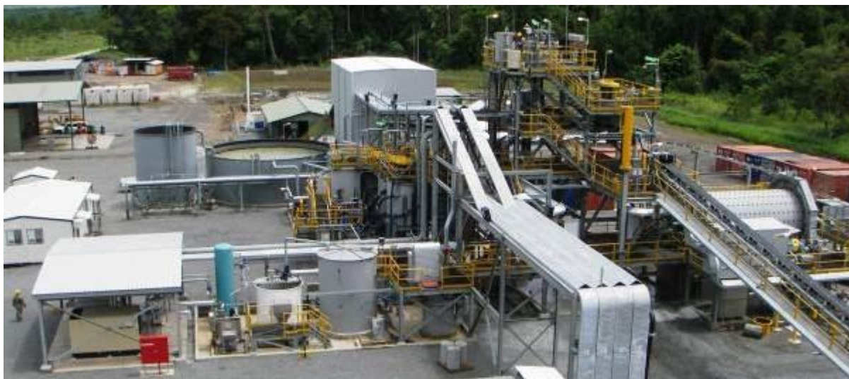
Figure 95: Photograph of the processing plant (2008)
