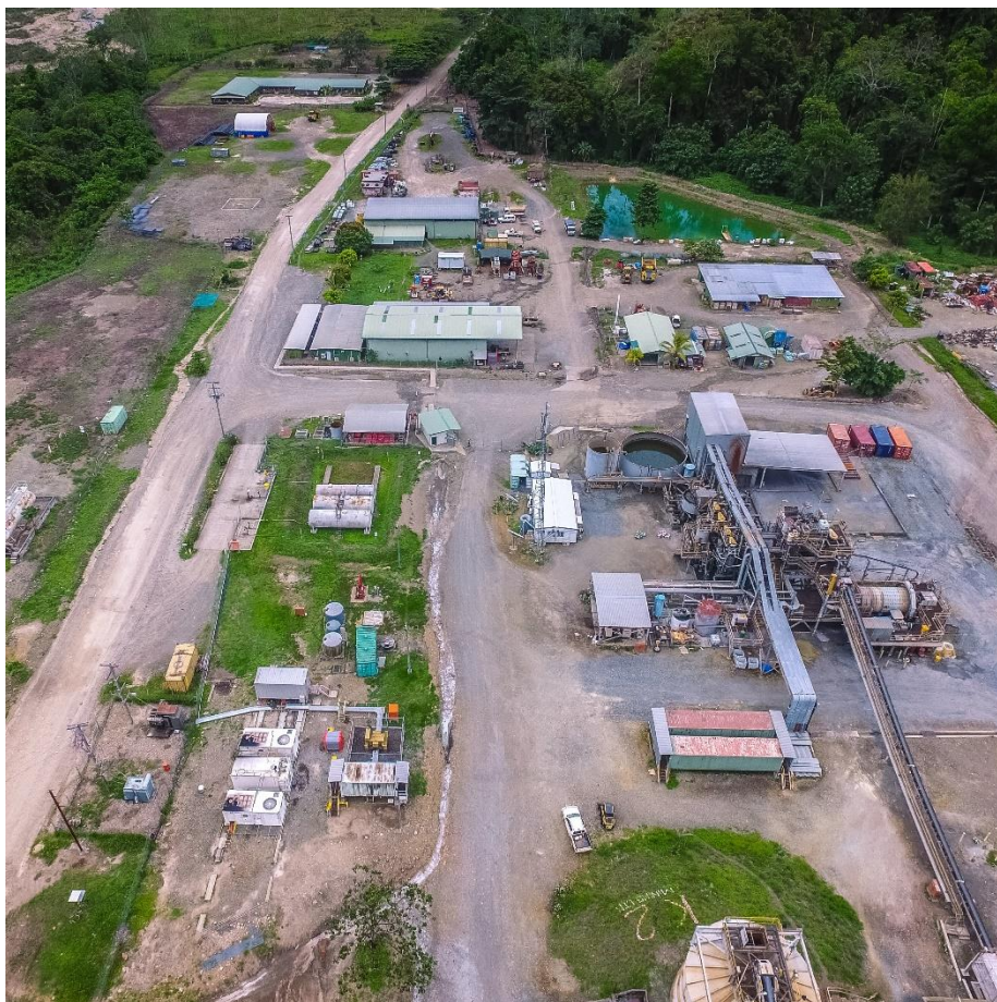
Figure 99. Oblique view of Process Plant and office infrastructure area (Nov 2017)
