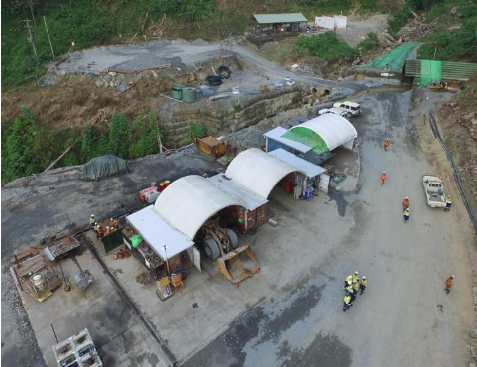
Figure 98: Aerial view of 800 Portal Infrastructure (June 2018)
