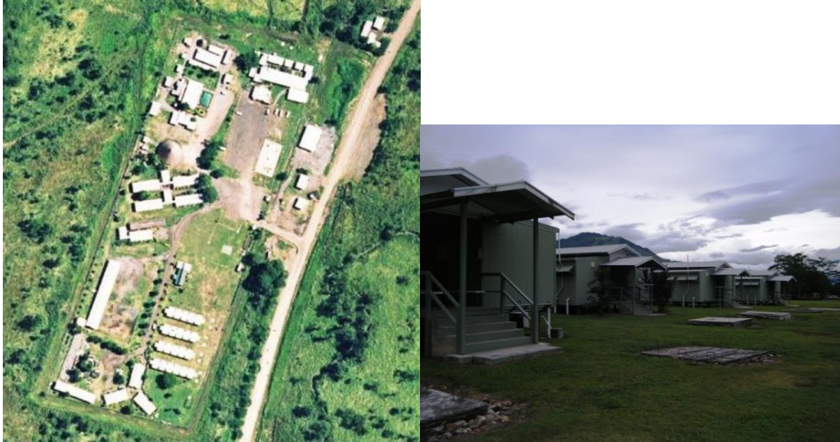
Figure 5 Aerial and Ground view of Kumian Accommodation Camp (circa 2009)
