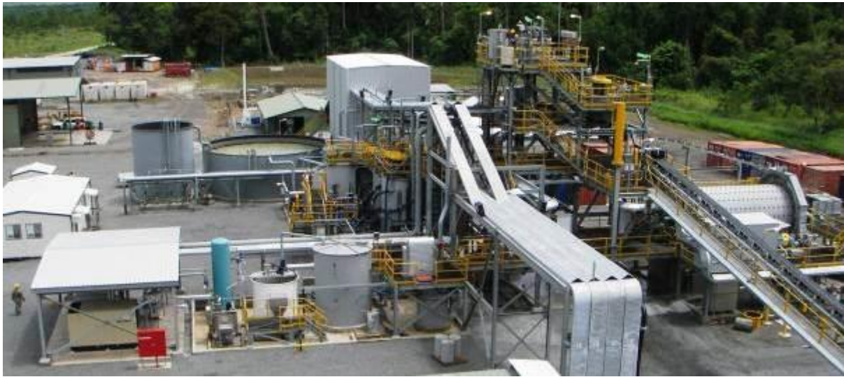
Figure 33: Photograph of the processing plant (2008)
