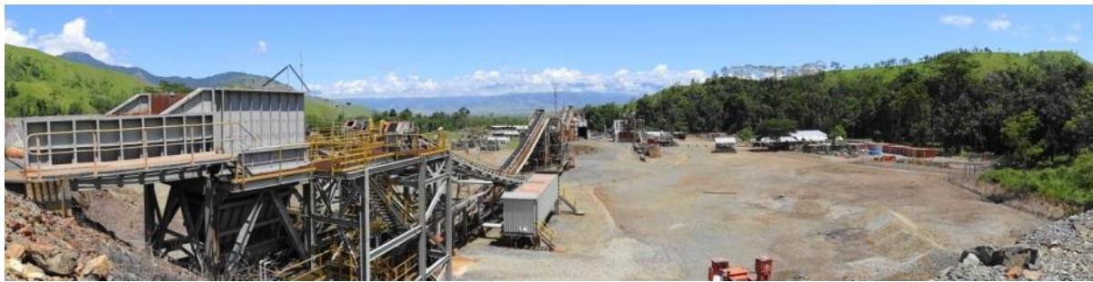
Figure 16: Photograph of the Crushing Circuit (2012)
