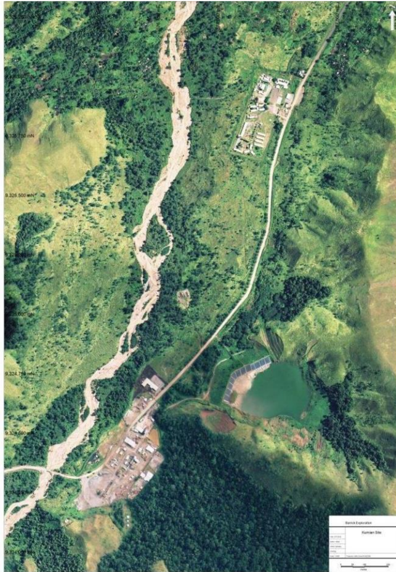
Figure 41. Aerial view of Process Plant, Tailings Storage Facility and Accommodation Camp (circa 2009) Source: Barrick 2012
