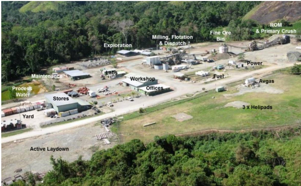
Figure 38. Oblique view of Process Plant and office infrastructure area (circa 2012)
