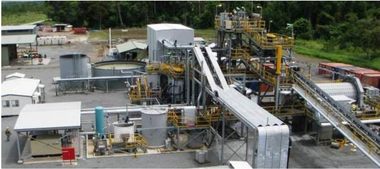
Figure 15: Photograph of the processing plant (2008)
