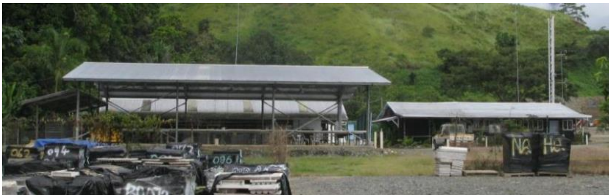
Figure 39. Profile view of Exploration Coreshed (left foreground), warehouse (left background) and offices (right foreground) (circa 2014)
