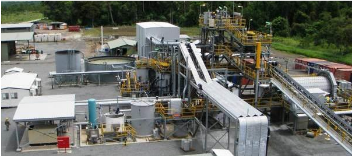
Figure 50: Photograph of the processing plant (2008)
