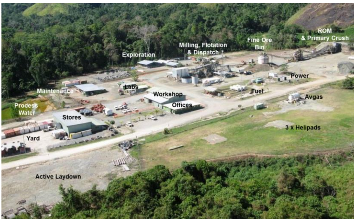
Figure 53. Oblique view of Process Plant and office infrastructure area (circa 2012)
