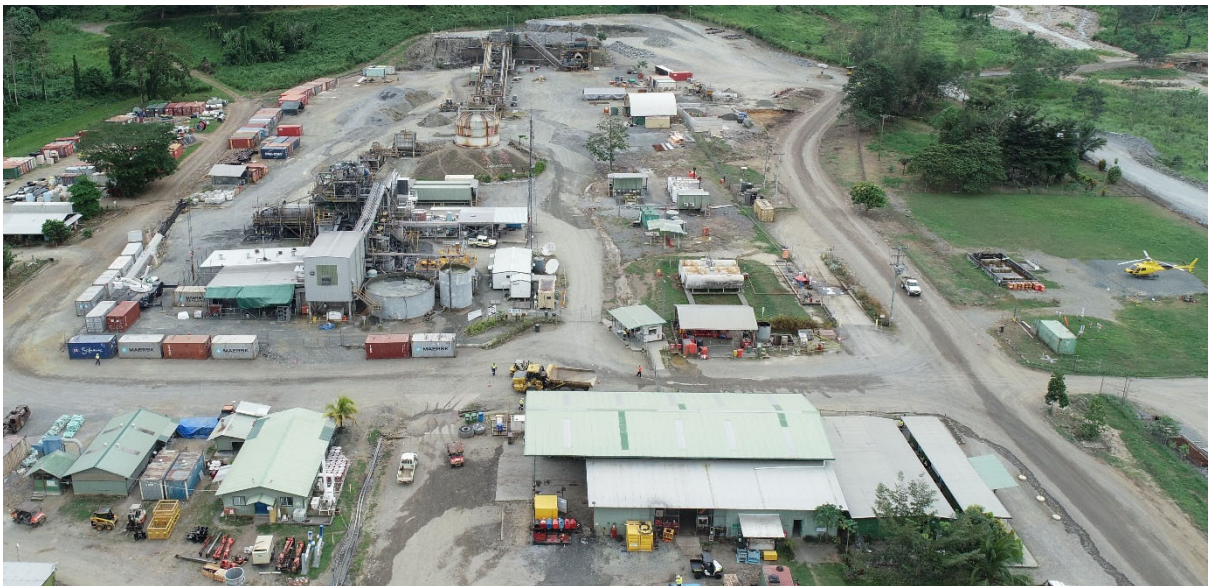
Figure 109. View of Process Plant and office infrastructure area (June 2020)
