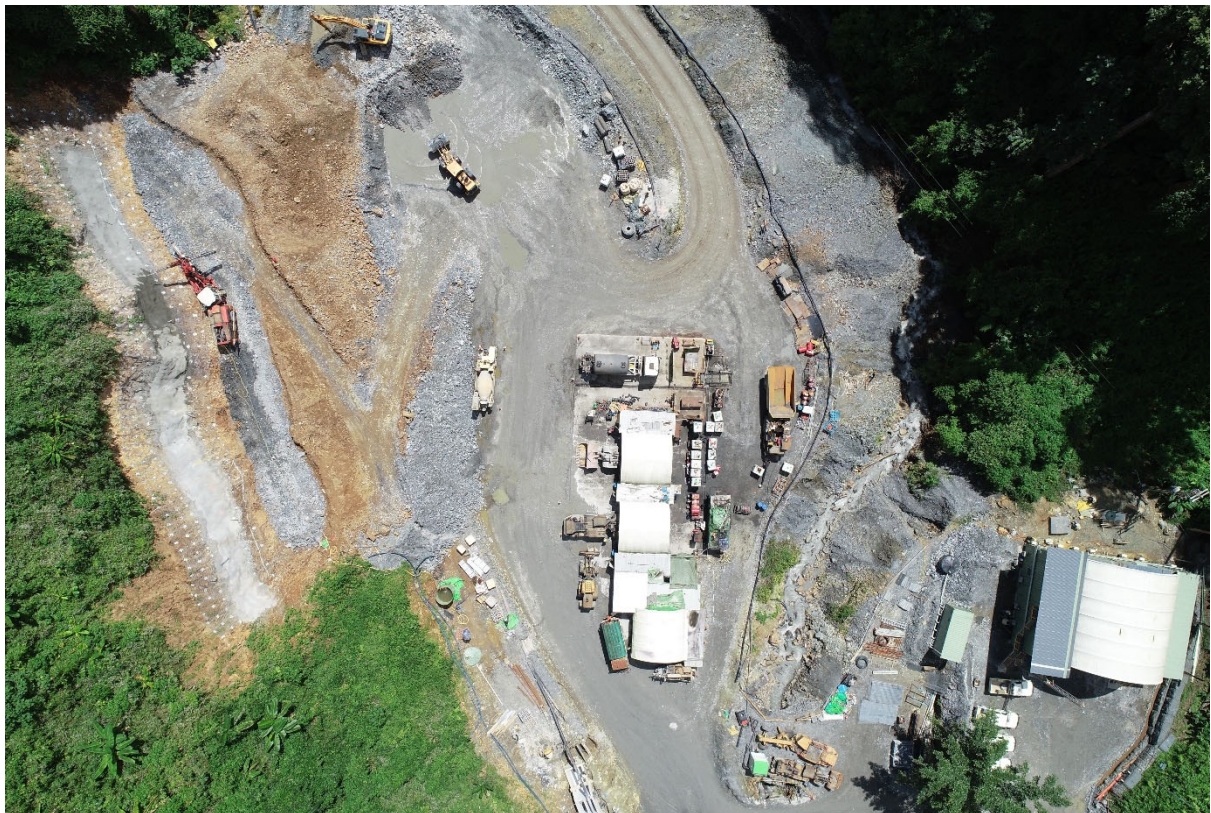
Figure 107. Aerial view of 800 Portal Infrastructure (July 2020)
