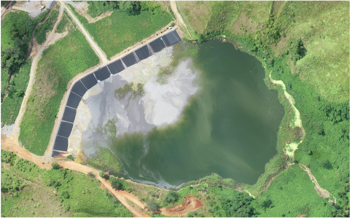
Figure 110. Aerial view of Tailings Storage Facility (May 2020)
