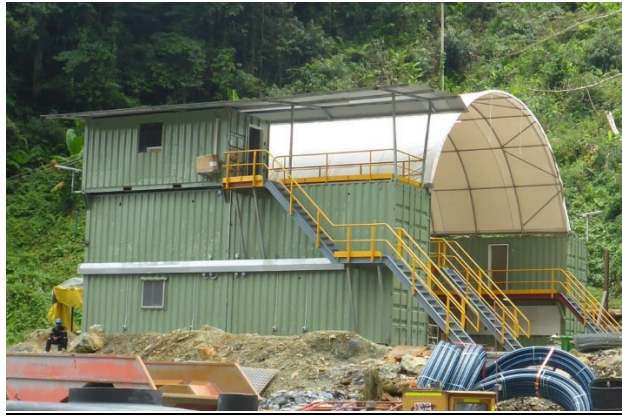
Figure 91. Mine Portal Workshop under construction
