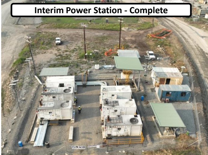
Primary Standby Power Station Phase 1 Expansion Complete (10.7 MW Prime Power Output (1) )
