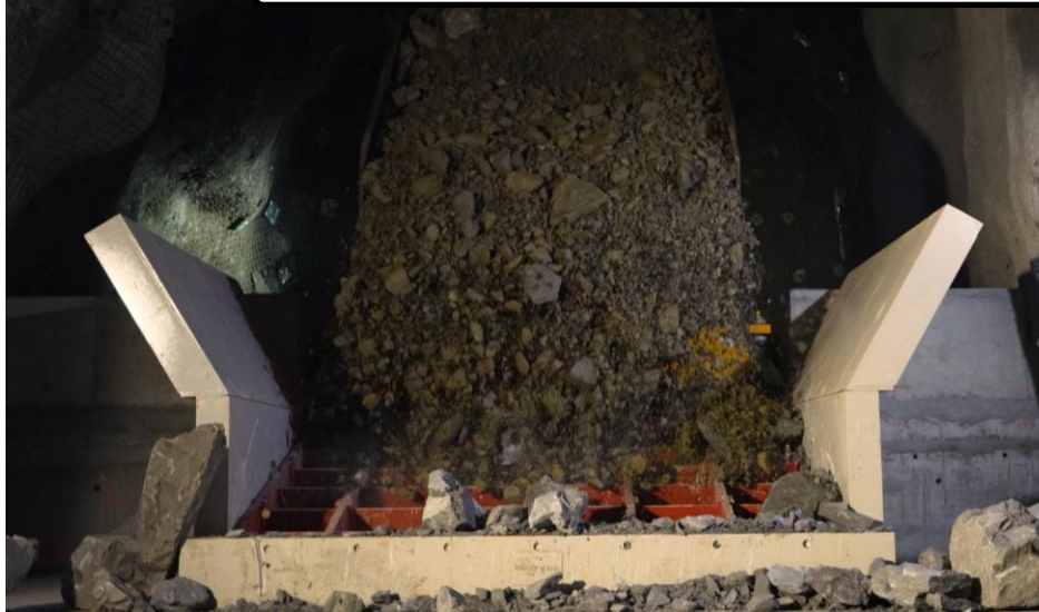
New Dedicated Ore and Waste Passes – Leveraging Mine's Gravity Advantage
