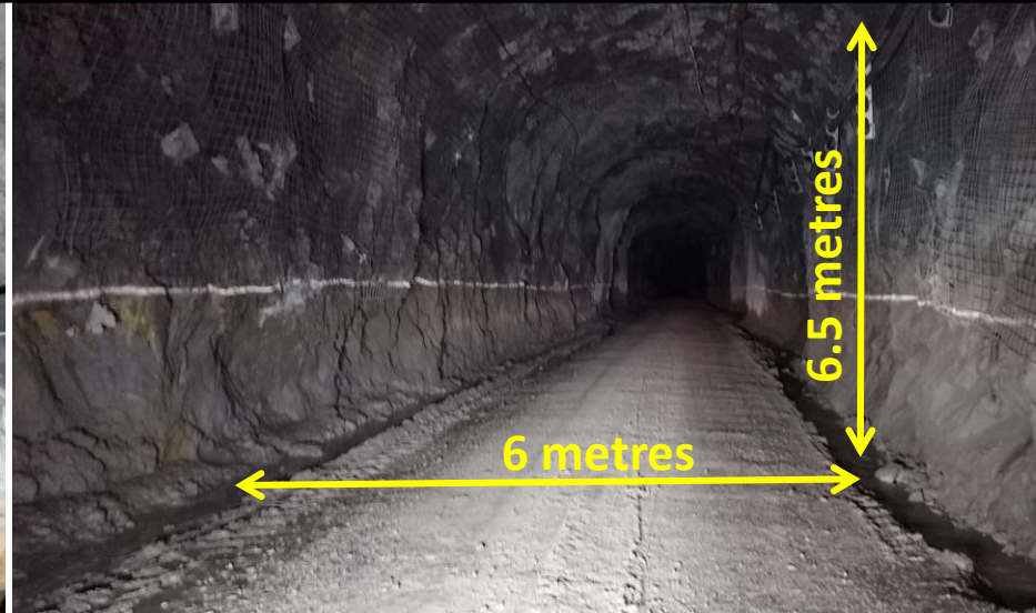
New Dedicated Ore and Waste Passes – Leveraging Mine's Gravity Advantage
