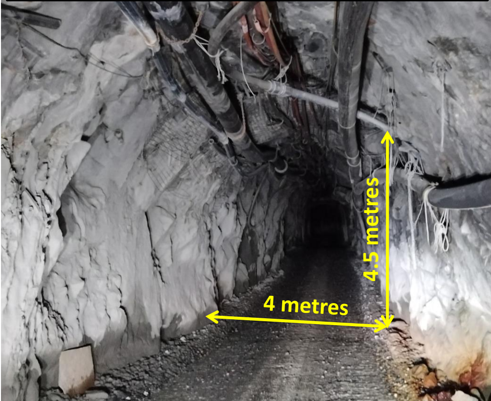
Existing Incline to Main Mine Transported 1 mt (waste & ore) in 2022
