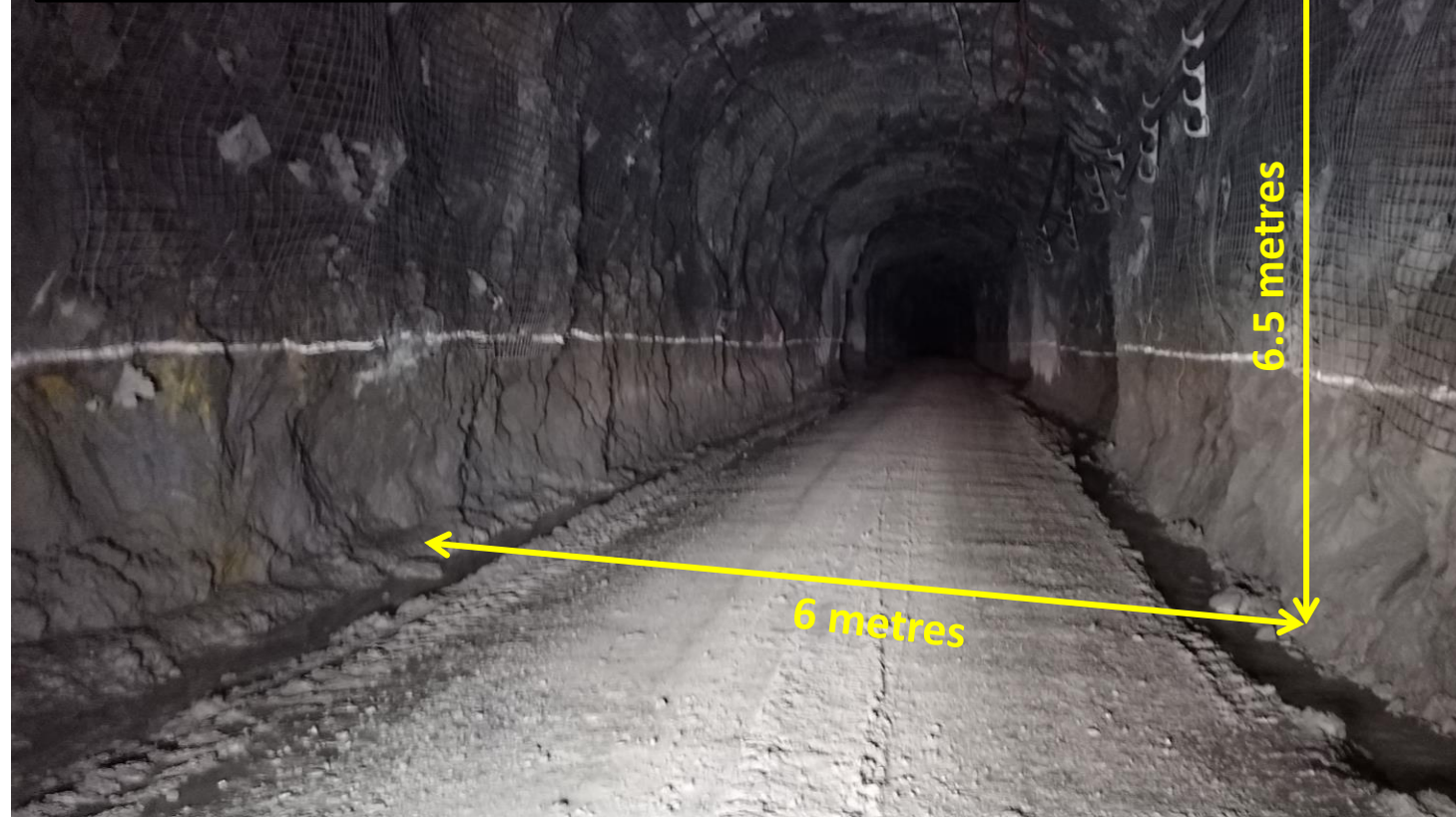
New Twin Incline (#2) Under Development High Speed, Large Travel way, Gradual Gradient
