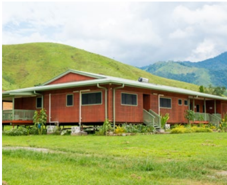
K92 training centre located at the Kainantu Gold Mine
